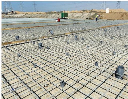
Jizan Flood Mitigation Channel Largest GFRP project in the world ©Mateenbar
