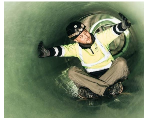
Water supply pipeline refit in Bełchatów, Poland. ©Saertex Multicom
